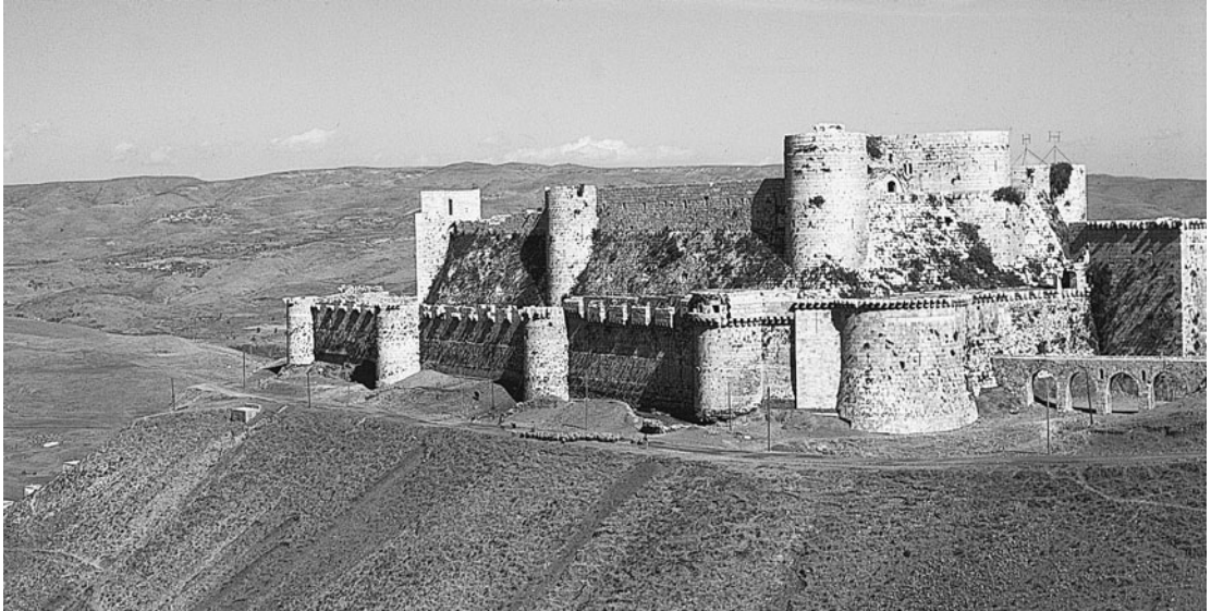
17. Krak des Chevaliers in Syria (in Arabic Hisn al-Akrad), one of the strongest and most aesthetically satisfying of the castles built by the Christian rulers of Outremer. Given to the Hospitallers in 1144, it fell to the Mamluks in 1271. In fact most Frankish forts were built away from exposed frontiers and acted as centres of administration and lordship.
